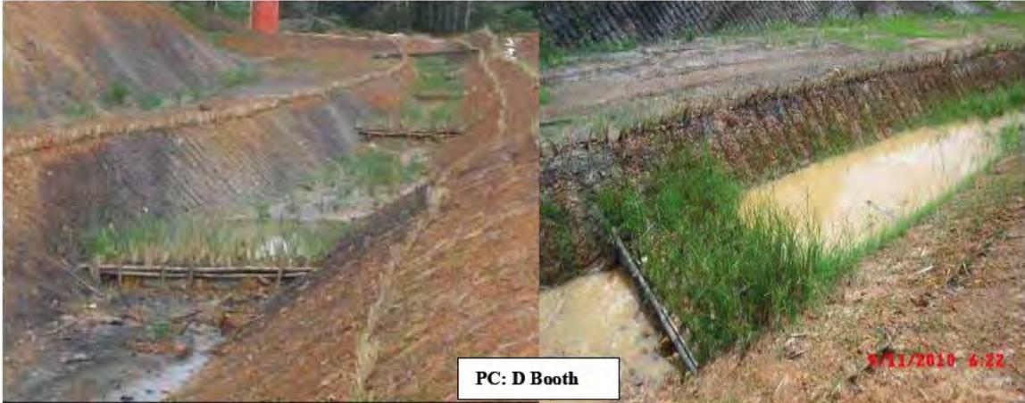
**Figure 59.** Vetiver planted for channel bank stabilization (along the channel) and sediment traps (cross the channel). Source: [www.vetiver.org](http://www.vetiver.org)
