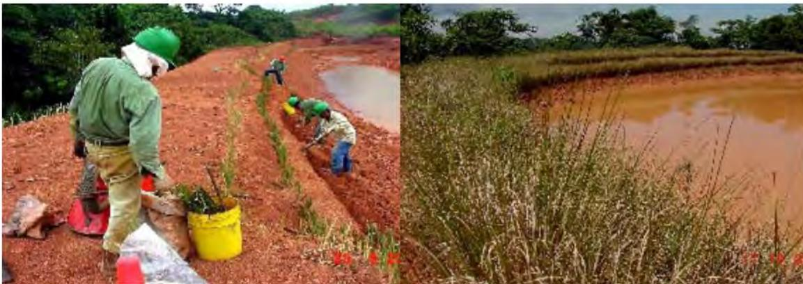
**Figure 65.** Vetiver planted for reinforcement of lagoon dikes (left) and 14 months after planting (right). Source: Luque et al., 2006.
