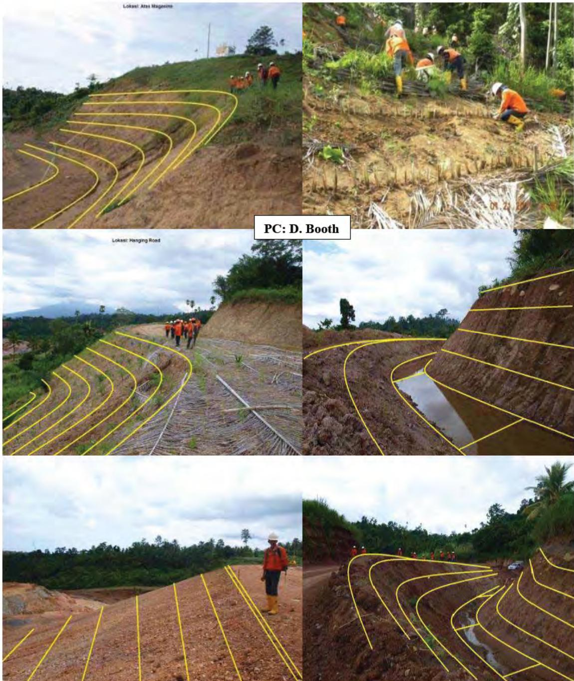
**Figure 48.** Design and application of Vetiver grass technology throughout extensive infrastructure and drainage. Source: [www.vetiver.org](http://www.vetiver.org).
