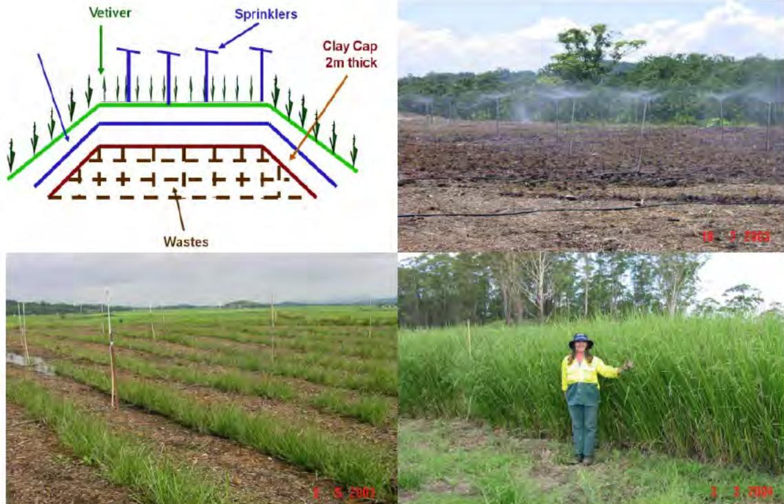
**Figure 35.** The Vetiver treatment at Stott Creek landfill mound: the diagrammatic cross section of the mound (top left), Vetiver irrigated every day with leachate after planting (top right), two (bottom left) and twelve (bottom right) months after planting.
