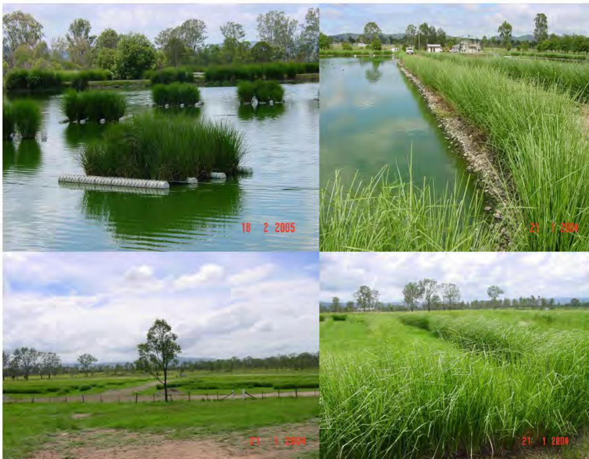
**Figure 23.** Vetiver treatment: hydroponic treatment (top) and ephemeral wetland with area of 1.5 ha (bottom).
