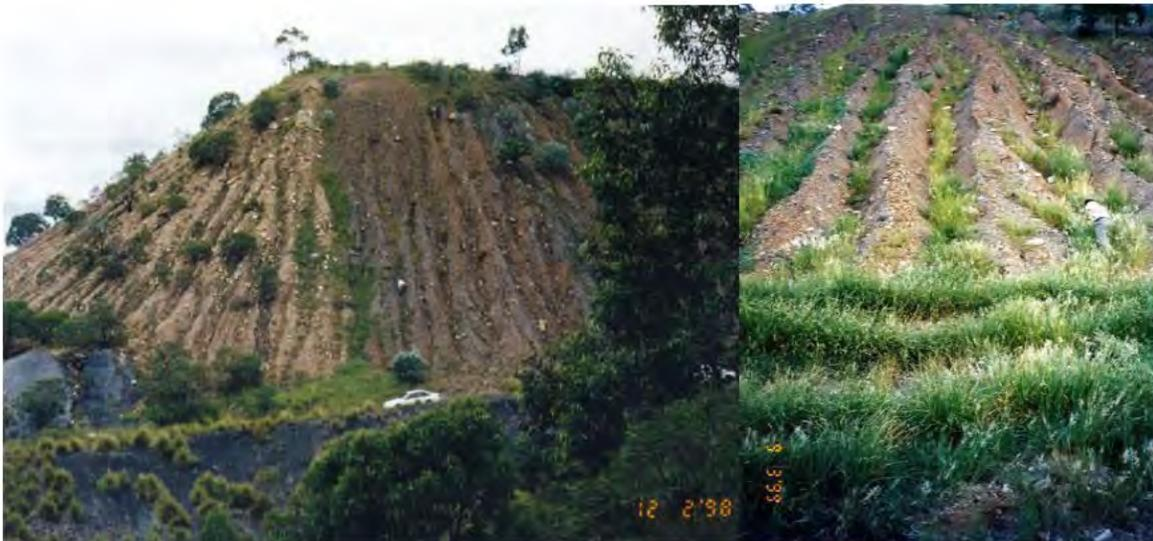
**Figure 54.** Old coal mine before (left) and after 1 year of planting Vetiver (right).
