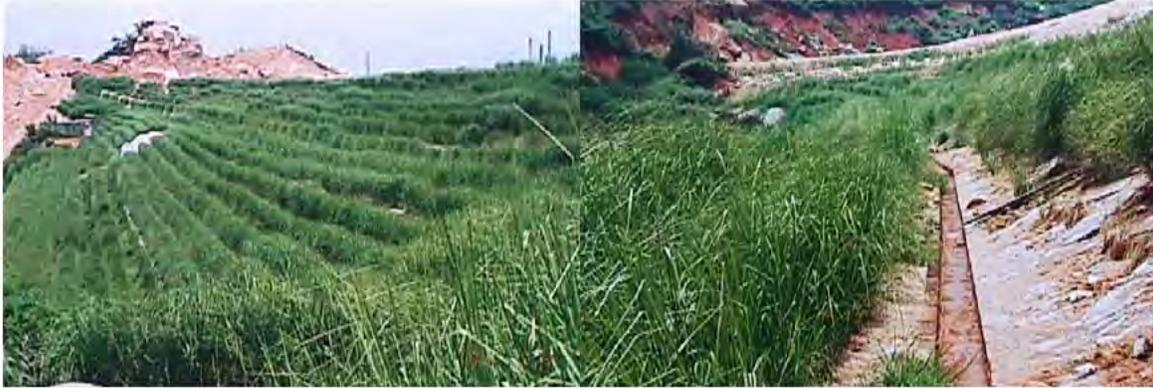
**Figure 41.** Vetiver planting on the slope of this old landfill mound in Guangzhou (left), leachate seepage was completely stopped one year after planting (right).
