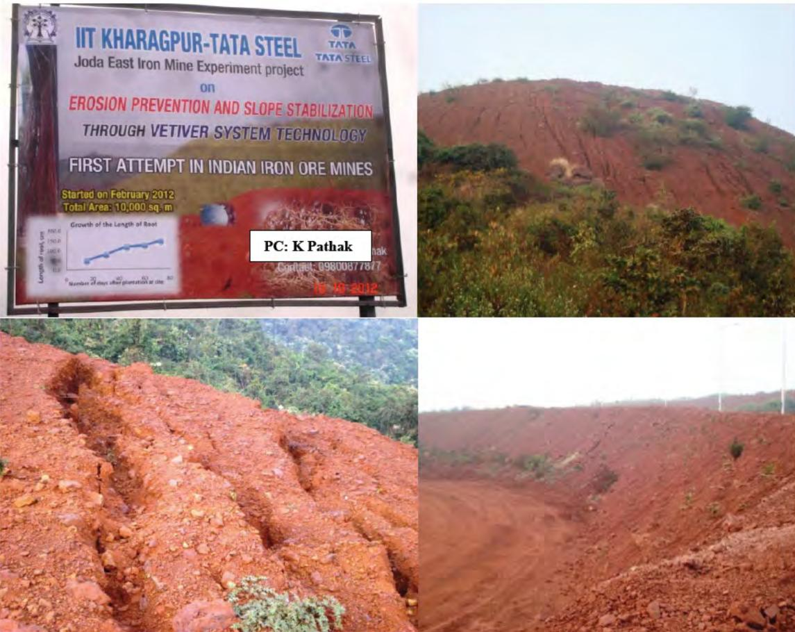
**Figure 76.** The old waste dump is highly erodible and steep (top and bottom left), and re-shaped to 40° (bottom right).
